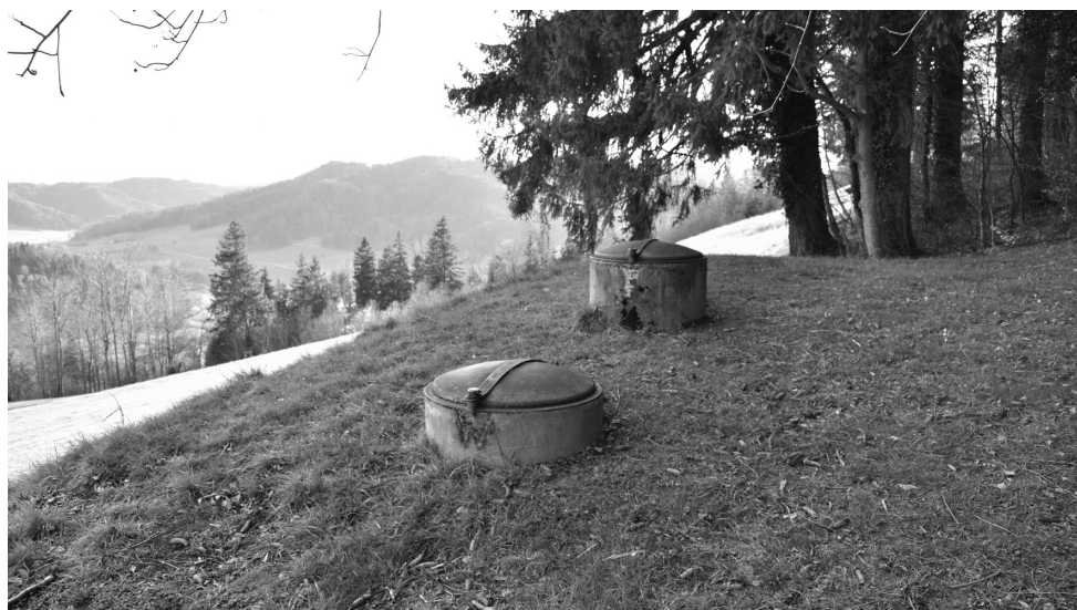
Reservoir Burstel Haselberg
