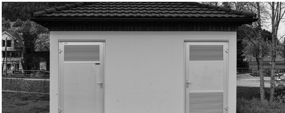
Transformatorstation Balterswilerstrasse Ifwil
